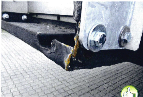
Lead in plate Correctly executed repair
